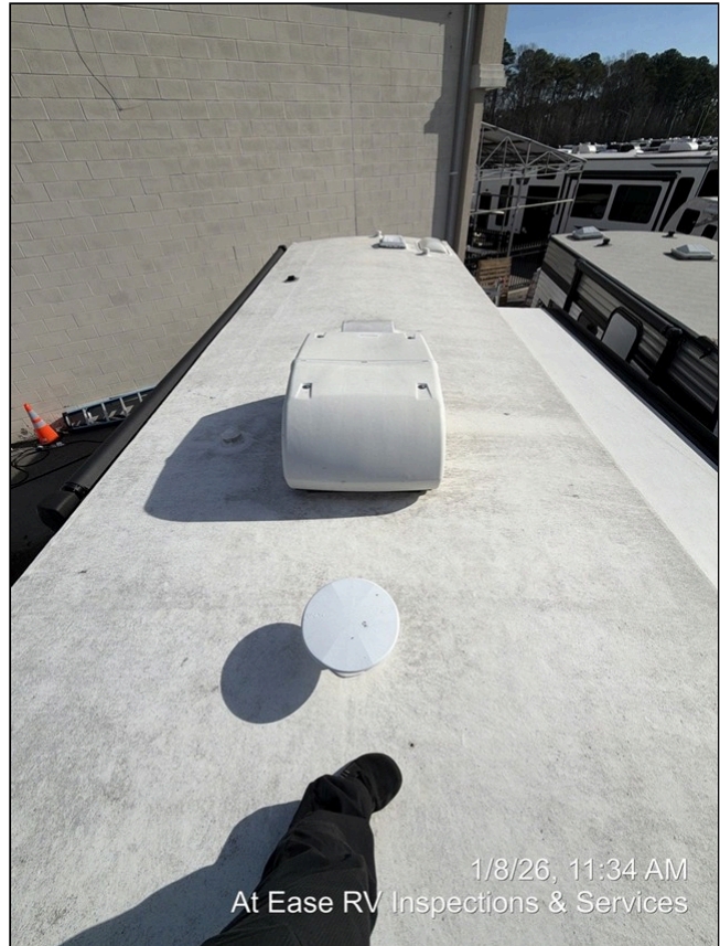
Front to back of roof
