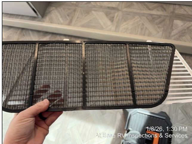
17.14 Item 1 (Picture) AC filter
