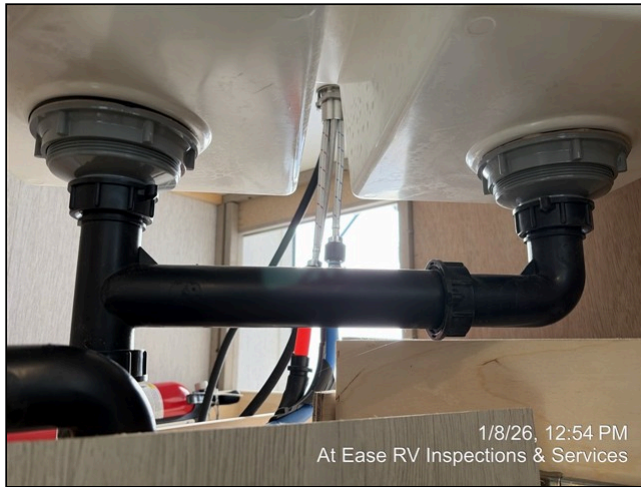
19.6 Item 1 (Picture) Under sink 1
