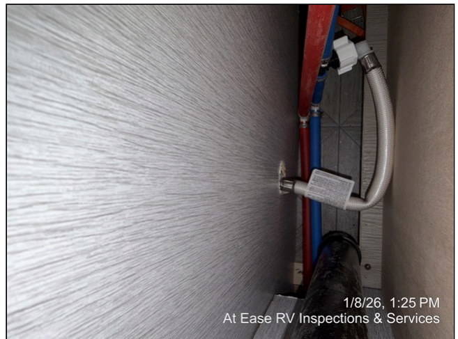
19.28 Item 2 (Picture) Looking down under bathroom sink
