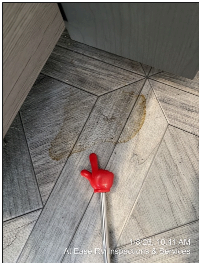
9.4 Item 2 (Picture) Stain on floor on front side of slideout
