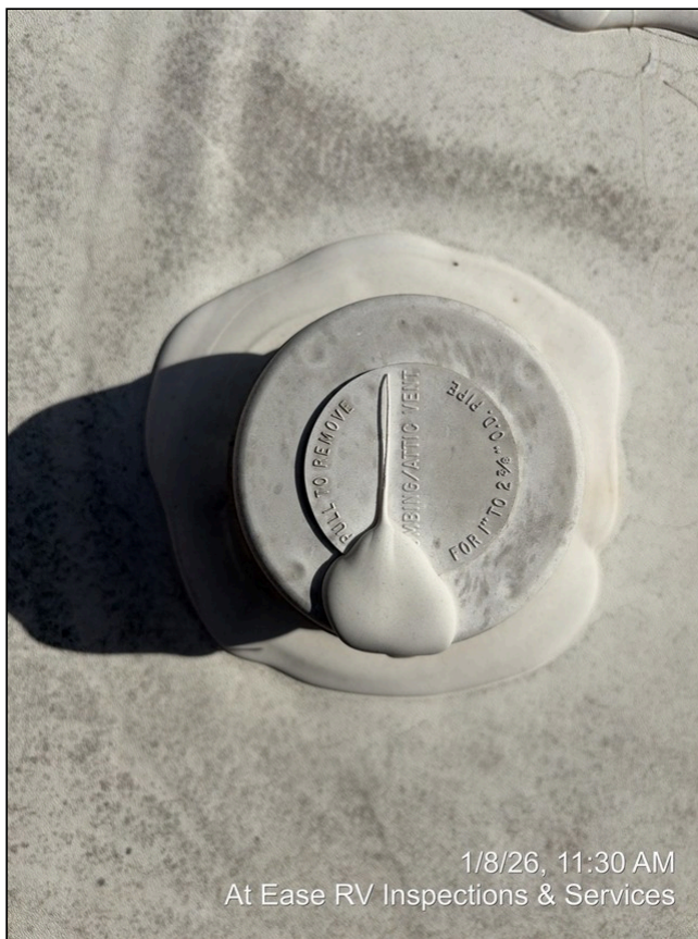
6.8 Item 1 (Picture) 1 of 3 plumbing vents
