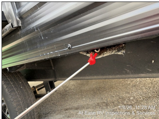
12.16 Item 1 (Picture) Gap in covering
