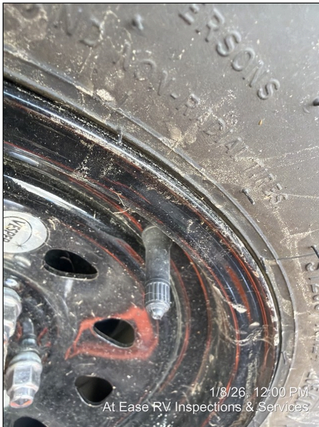
10.3.B Item 1 (Picture) Valve extension
