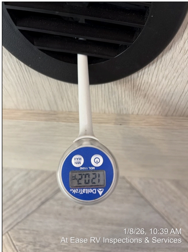
17.10 Item 1 (Picture) Vent under microwave
