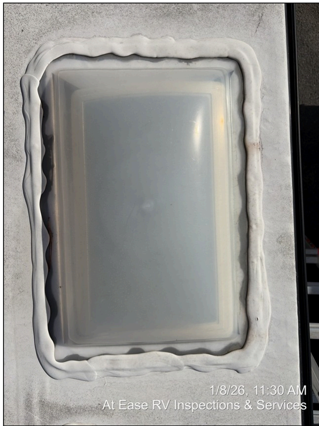
6.10 Item 1 (Picture) Skylight
