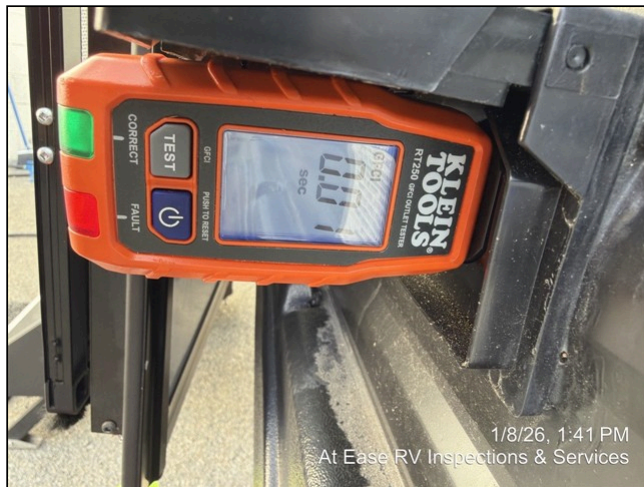
14.11 Item 1 (Picture) GFCI testing
