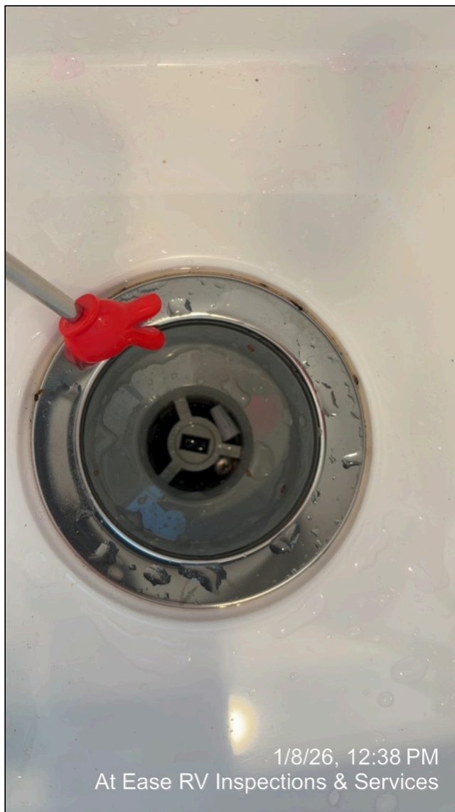
19.3 Item 1 (Picture) Wire cap and screw in drain
