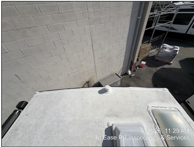
6.3 Item 1 (Picture) Rear wall joint
